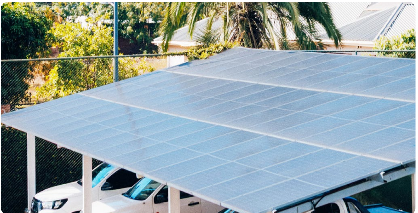
Solar energy powering the Commission's data centre, reducing reliance on the national grid.
